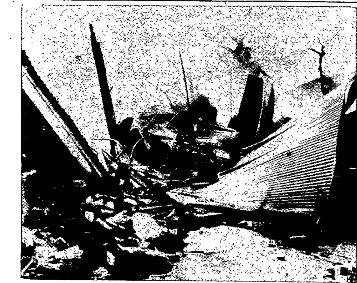
JAP BOMBERS PASSED OVER—Japanese bombers roared over Honolulu December 7 in a surprise attack and left this wrecked corner. It once was a thriving business district, but incendiary bombs set a fire that destroyed 20 buildings.
